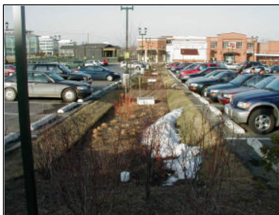
Bioretention Cell Source: LID Center
