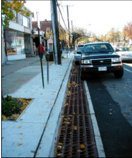
Gutter filter in Mount Rainier, MD Source: LID Center
