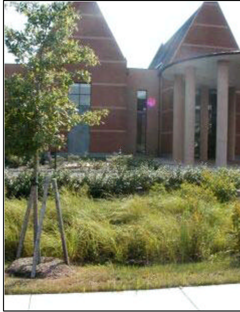
Native vegetation in bioretention cell at Alexandria Central Library
