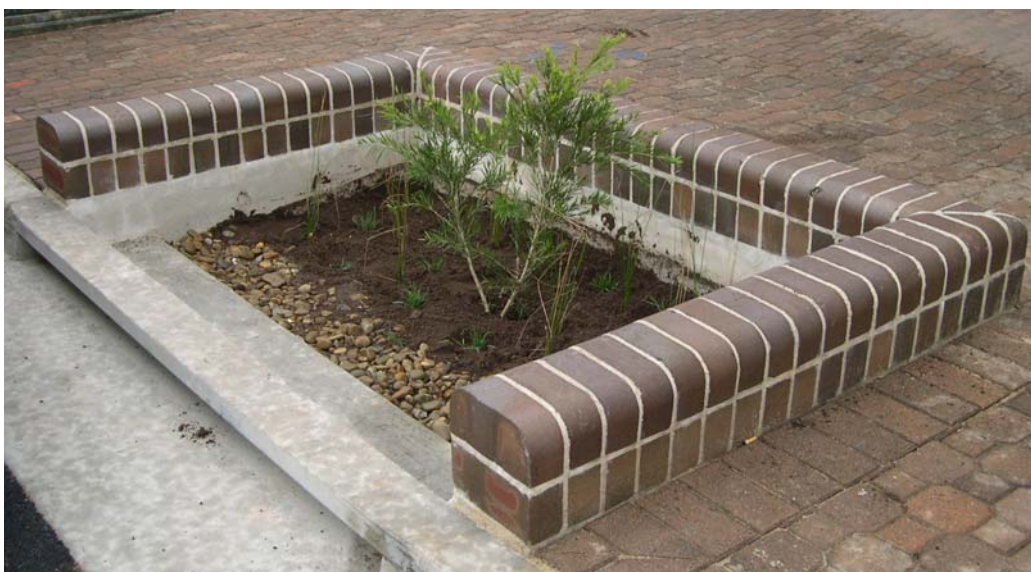
Plate 1 Street Tree Planter Bioretention System, Normurra Avenue Water Sensitive Urban (art work not installed at time of photo)
