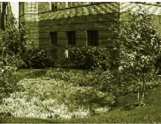
Above: This bioretention cell at a office park also helps to fulfill site landscaping requirements. Photo: Low Impact Development Center
