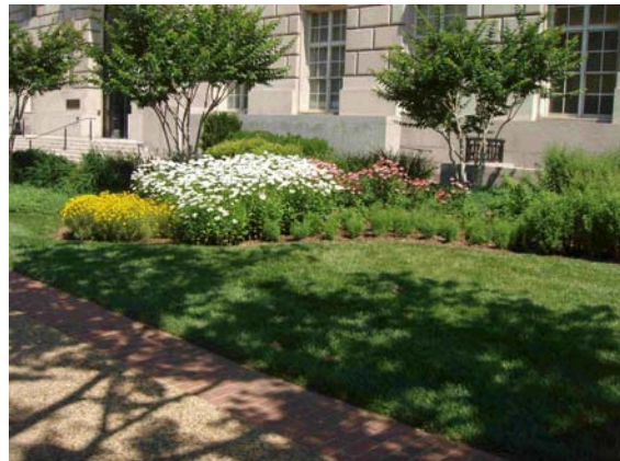
Bioretention Cell at US EPA Headquarters
